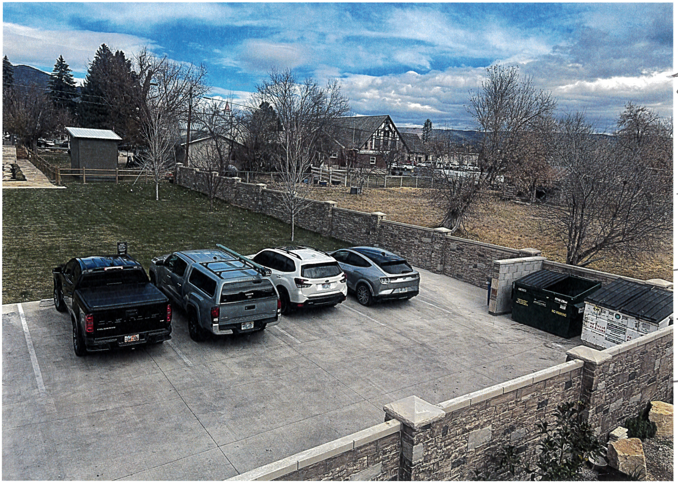
North Side Property
